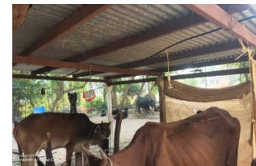
Installed cooling spray for animals in association with C. C. Patel Community Science Centre, SPU
